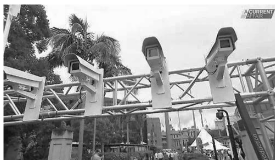
Figure 1: Photo of CCTV cameras.
