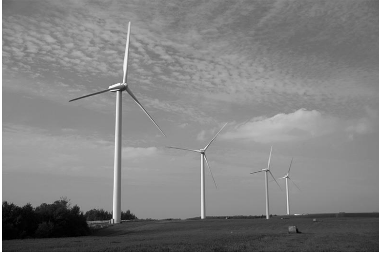
Figure 17: Photo of four (4) wind turbines at a wind farm.
